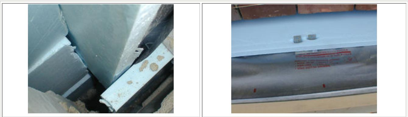
*Improperly installed rigid foam boards leave gaps in the thermal and air barrier assemblies.*
