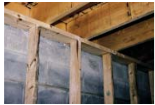
Photograph 1 Interior stud framing located at basement perimeter
