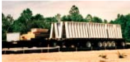
Photograph 10 Pre-cast basement walls
