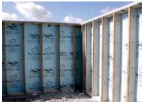
Photograph 11 Pre-cast basement walls with XPS foam insulation
